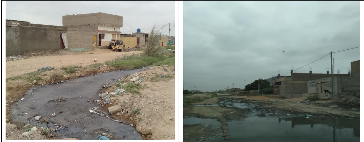
Figure 5-16: Existing condition of Sewerage system at the sub-project location
