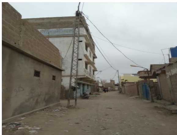
Existing condition of road at haji Abdul Karim Mohla
