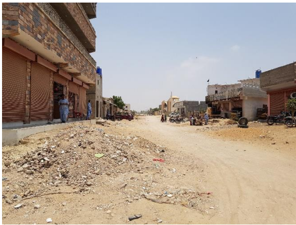
Existing condition of paka sarak road
