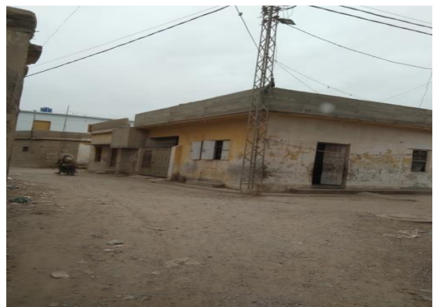
Existing condition of road at haji Abdul Karim Mohla
