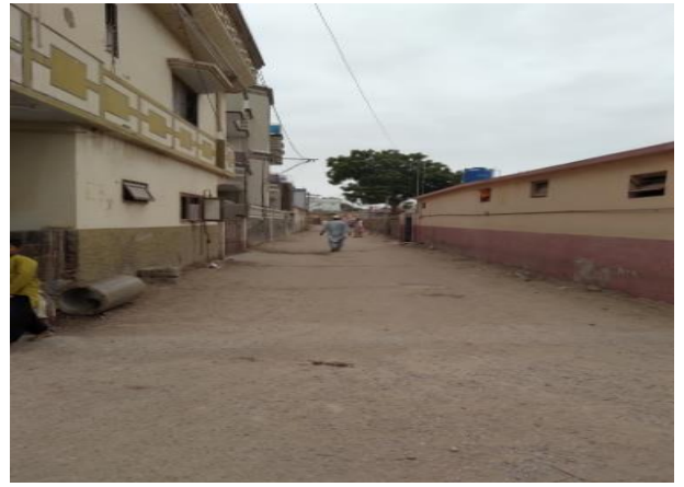
Existing condition of road at Haji Shafi Mohammad Mohla
