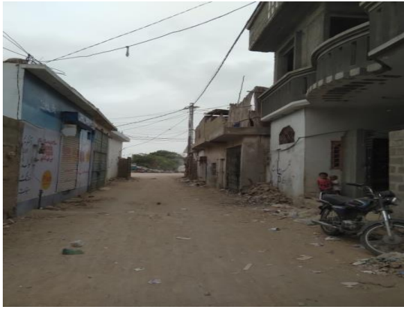
Existing condition of road at Haji Shafi Mohammad Mohla
