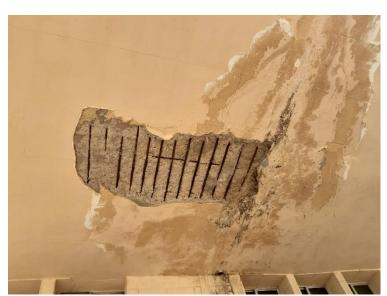
Spalling of concrete at bottom and seepage can be se
