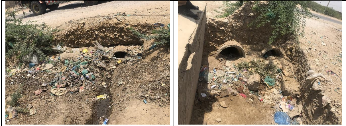
Figure 5-11: Existing condition of culverts at the sub-project location
