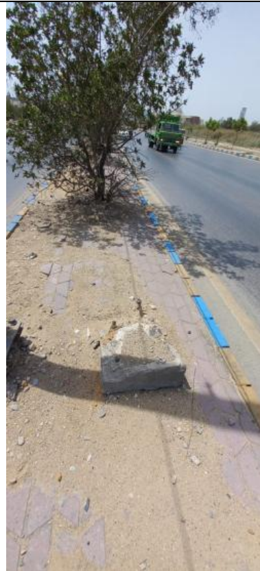
Missing Pole of Existing street Light
