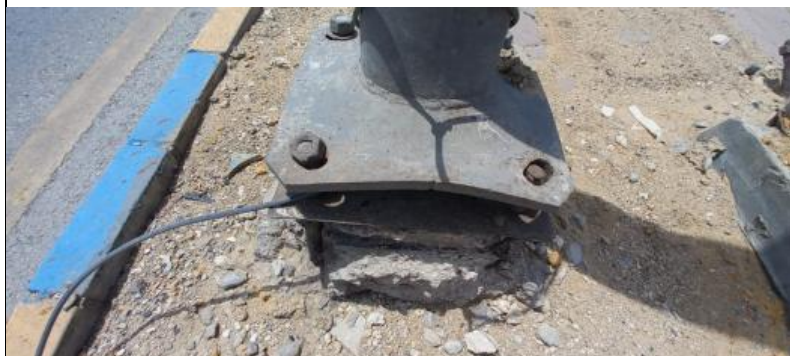
Damaged foundation of pole
