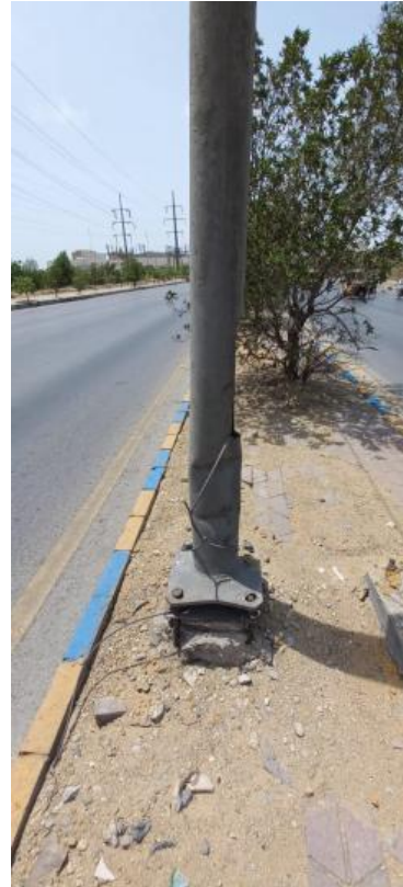
Rusted pole of existing Street Lights
