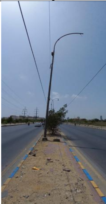
Missing lights from pole and also little tilted
